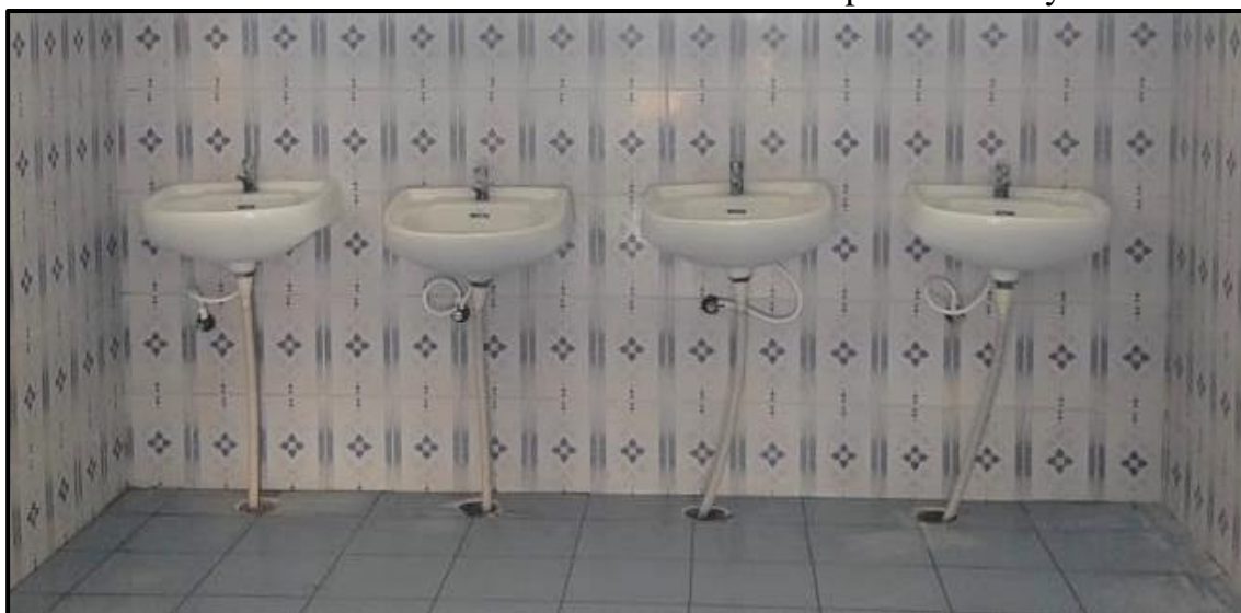
Proper Maintenance of Taps without leakages in Seshadri Rao Gudlalleru Engineering College, Andhra Pradesh.
