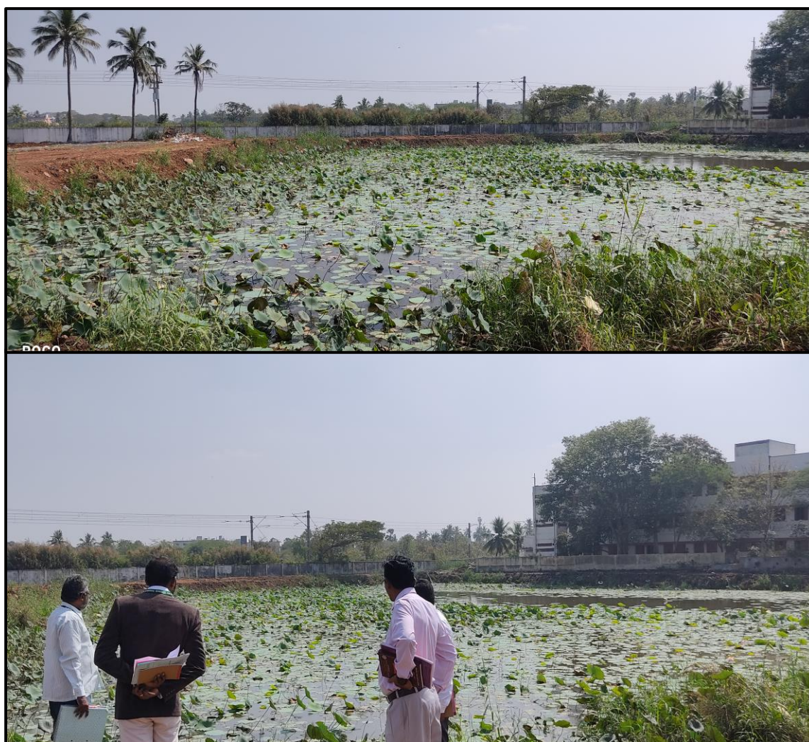
Percolation Pond in Seshadri Rao Gudlavalleru Engineering College, Andhra Pradesh.
